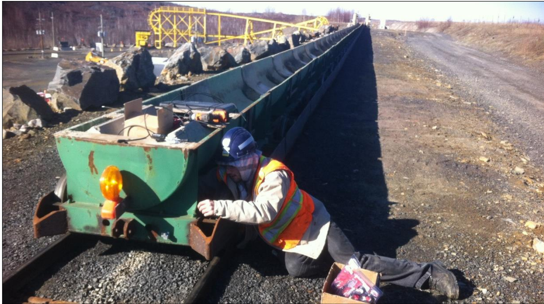
Figure 1-4: The Rail-Veyor® demonstration site used for in-situ data collection is situated in Sudbury, Ontario, Canada.
