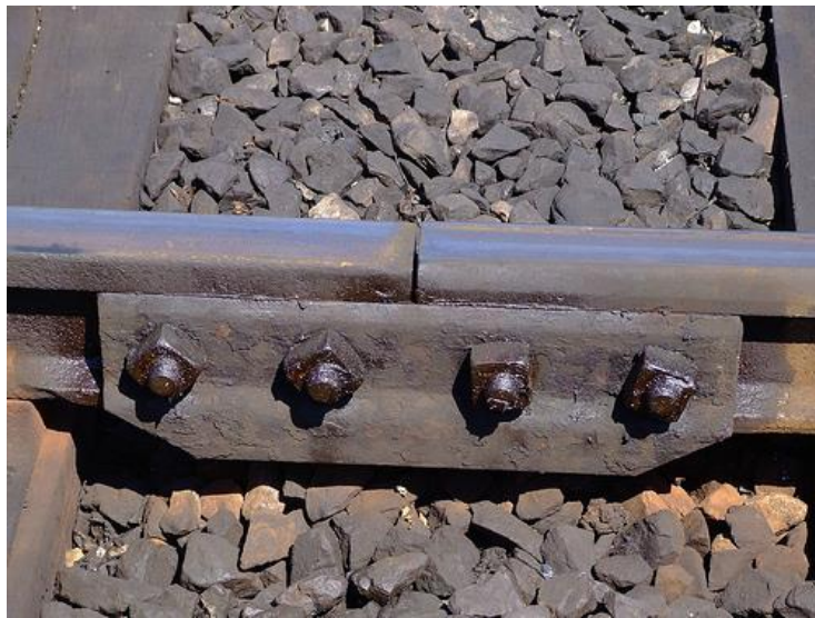
Figure 2-8: Fishplates Join Rail Sections (taken from [21])
